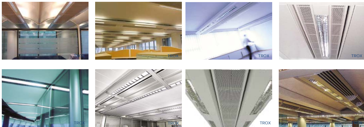
Figure 12: Examples of Multi-Service Chilled Beams
